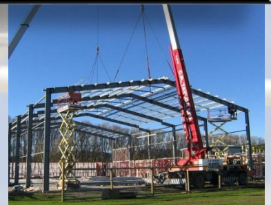
Erection of steel structures
