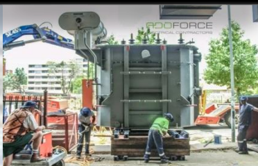
Installation of Equipment
